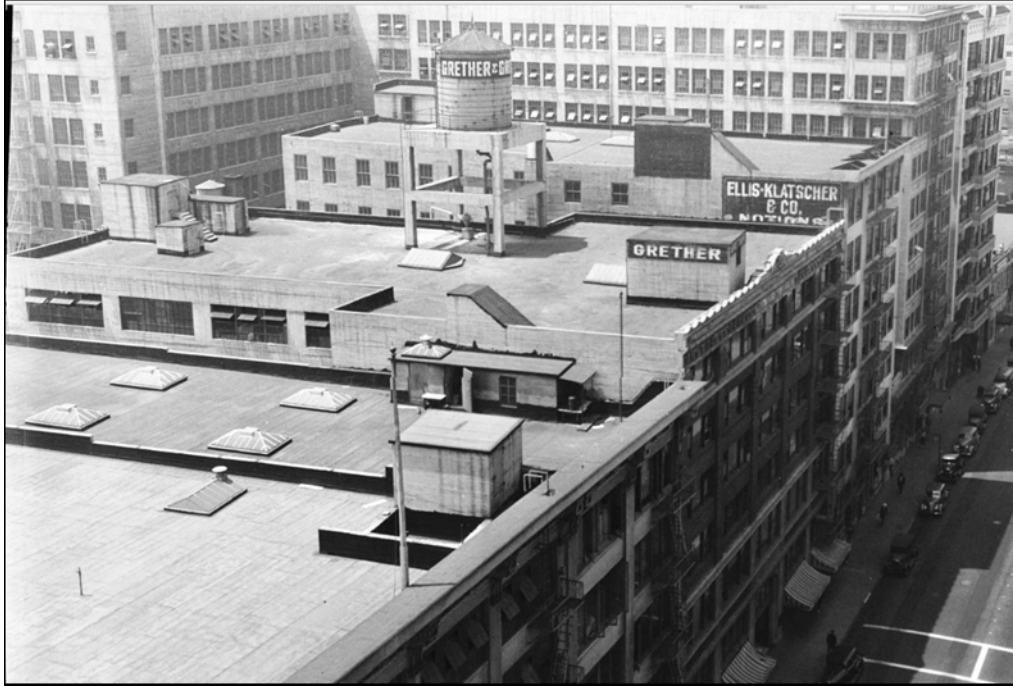
Figure 5 Grether & Grether Building (facade and rooftop) c. 1927 (USC Libraries Special Collections)
